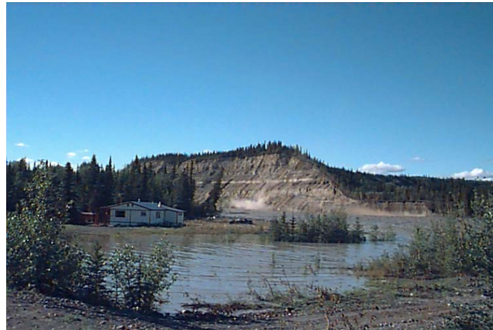
Photo 3: Home in foreground is upstream and on the south side of the Tazlina River Bridge, photo courtesy of Michael L. Bird, November 14, 1998.
